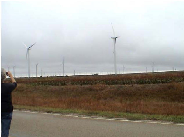
Wind Turbines located on The Smokey Hills Wind Farm
